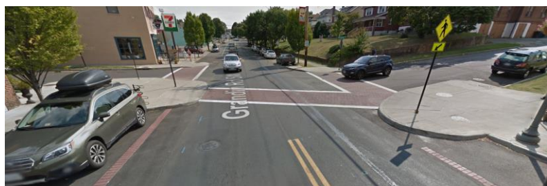
FIGURE 6. BULB-OUTS AT THE INTERSECTION OF GRANDIN ROAD SW AND WESTOVER AVENUE SW IN ROANOKE, VA.
