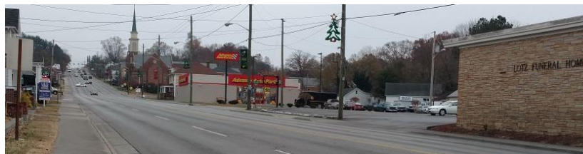
FIGURE 7. VIRGINIA AVENUE (TOP), BYPASS ROAD (MIDDLE), AND WASHINGTON AVENUE (BOTTOM).
