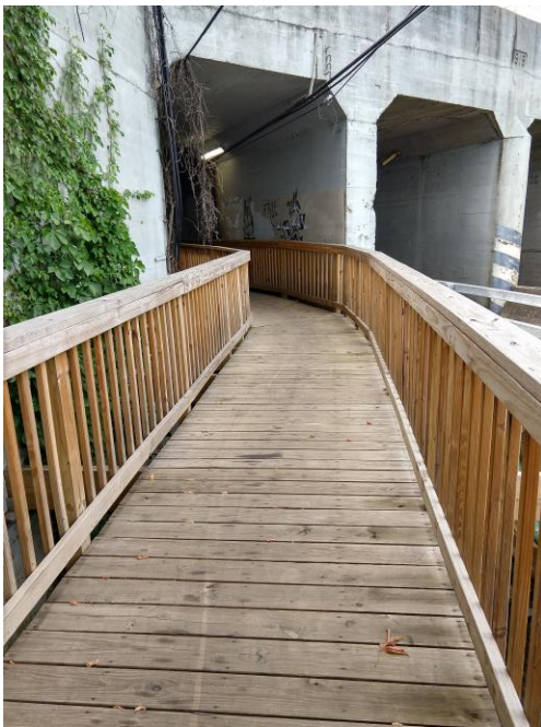
Figure 1. Facing south at the location of the counter
