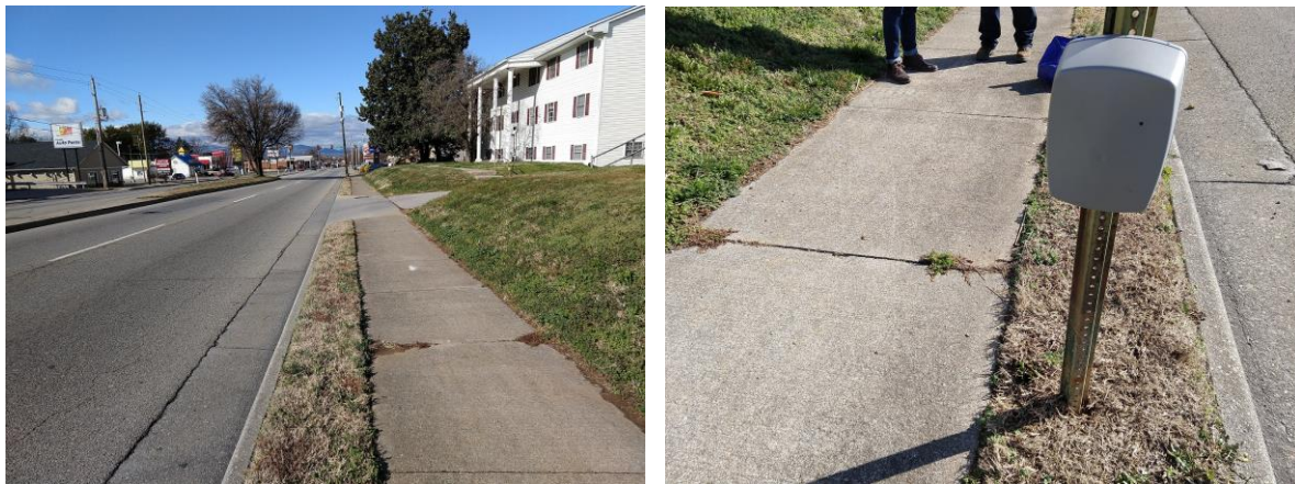
Figure 2. Location of counter. Left: Standing on the north side of Hardy Road facing east. Right: Facing west.
