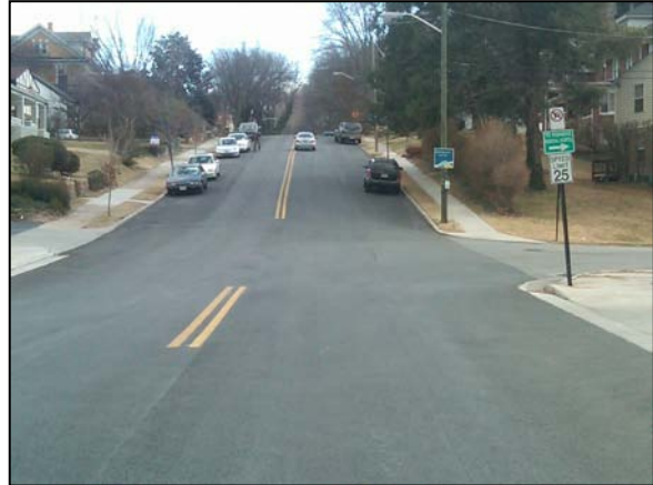
Center line shifted and downhill travel lane narrowed to install wide travel lane in uphill direction on Walnut Avenue/Mill Mountain Greenway (City of Roanoke)
