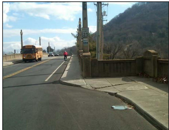
Wide travel lane with an "urban shoulder" on Walnut Avenue/Mill Mountain Greenway
