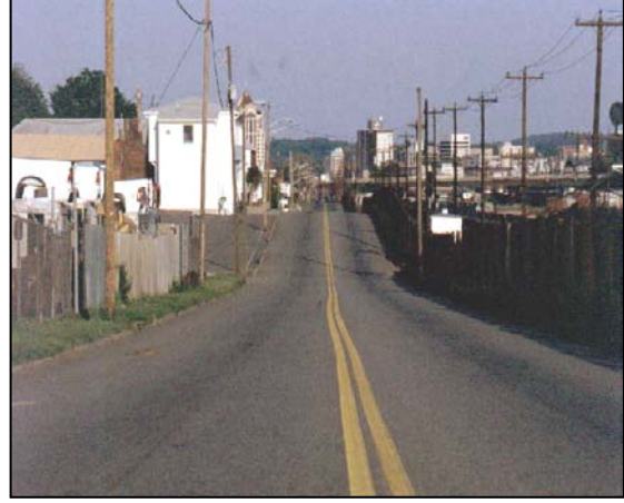
Wide travel lanes on Shenandoah Avenue prior to installation of bicycle lane
