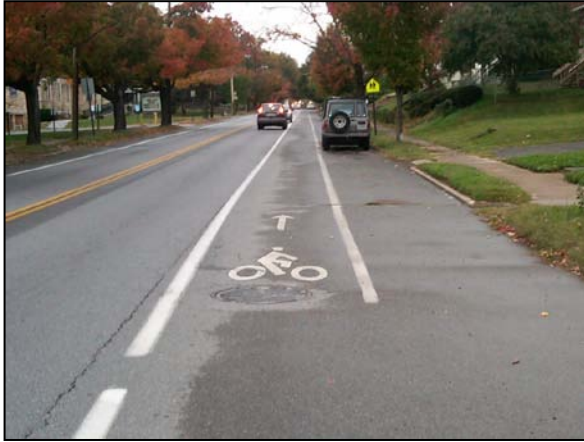
Bicycle lane on Memorial Avenue (City of Roanoke) installed as part of a "road diet" in 2000
